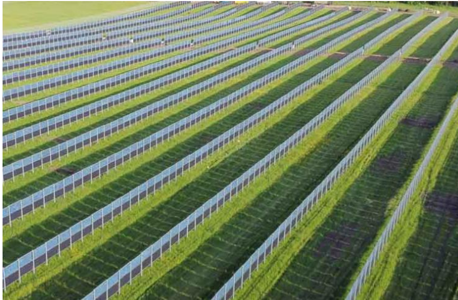
Figure 2: Next2Sun Agri-PV System ( image source: Next2Sun )
